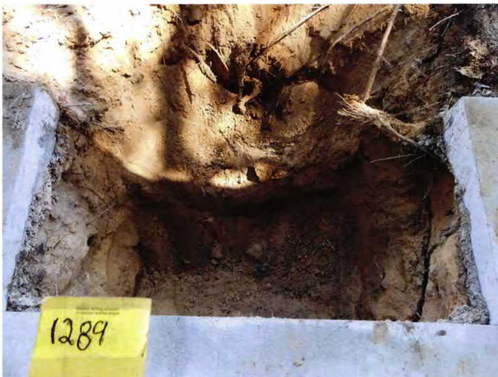
Picture 2: UST 1289Eagle excavation.
